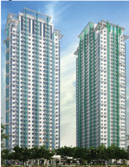
Figure 79: Manhattan Plaza Towers
