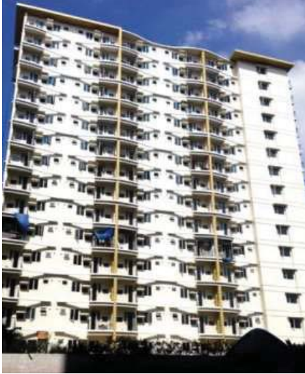
Figure 80: Palm Beach Villas Boracay Tower
